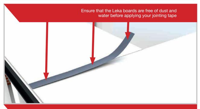
Ensure that the Leka boards are free of dust and water before applying your jointing tape
